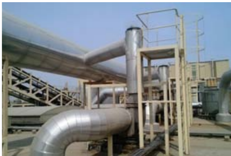
Recovery of steam from dryers - Lianyungang (China)
